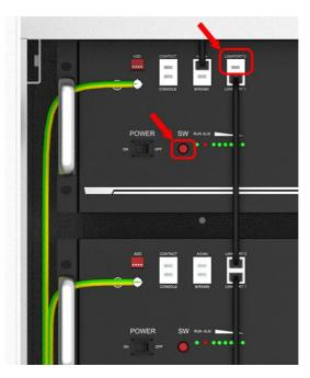
3) Press the **red SW button** of **master battery** to power on, all the battery LED light will be on one by one from the Master battery:
